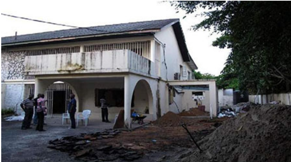
Transcorp Office under Renovation
