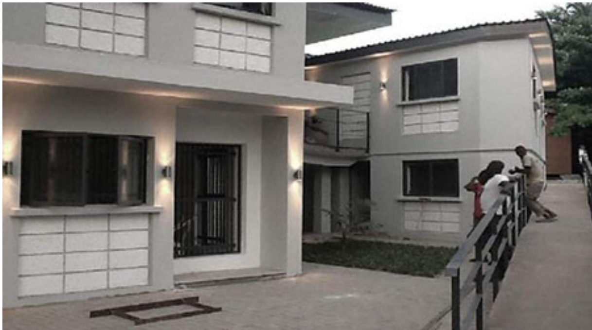
Avon Medical Hospital After Renovation
