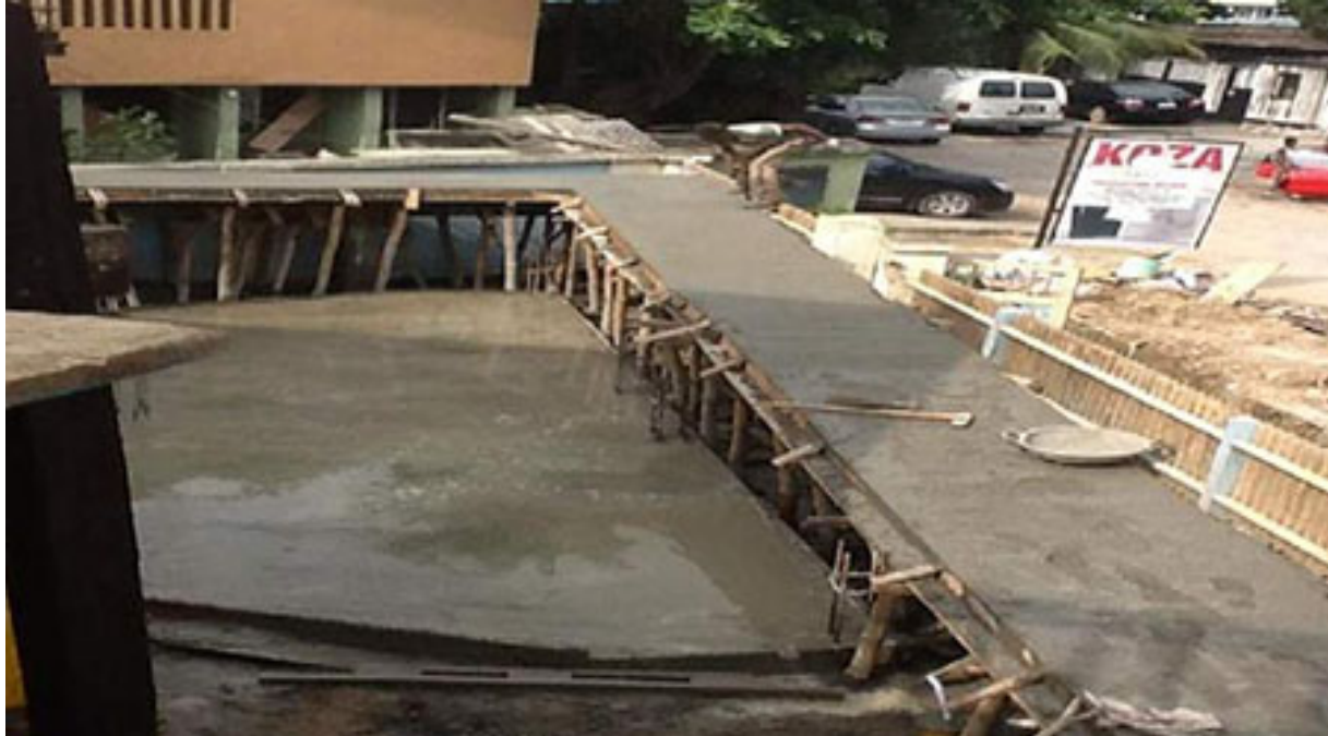
Avon Medical Hospital before Renovation
